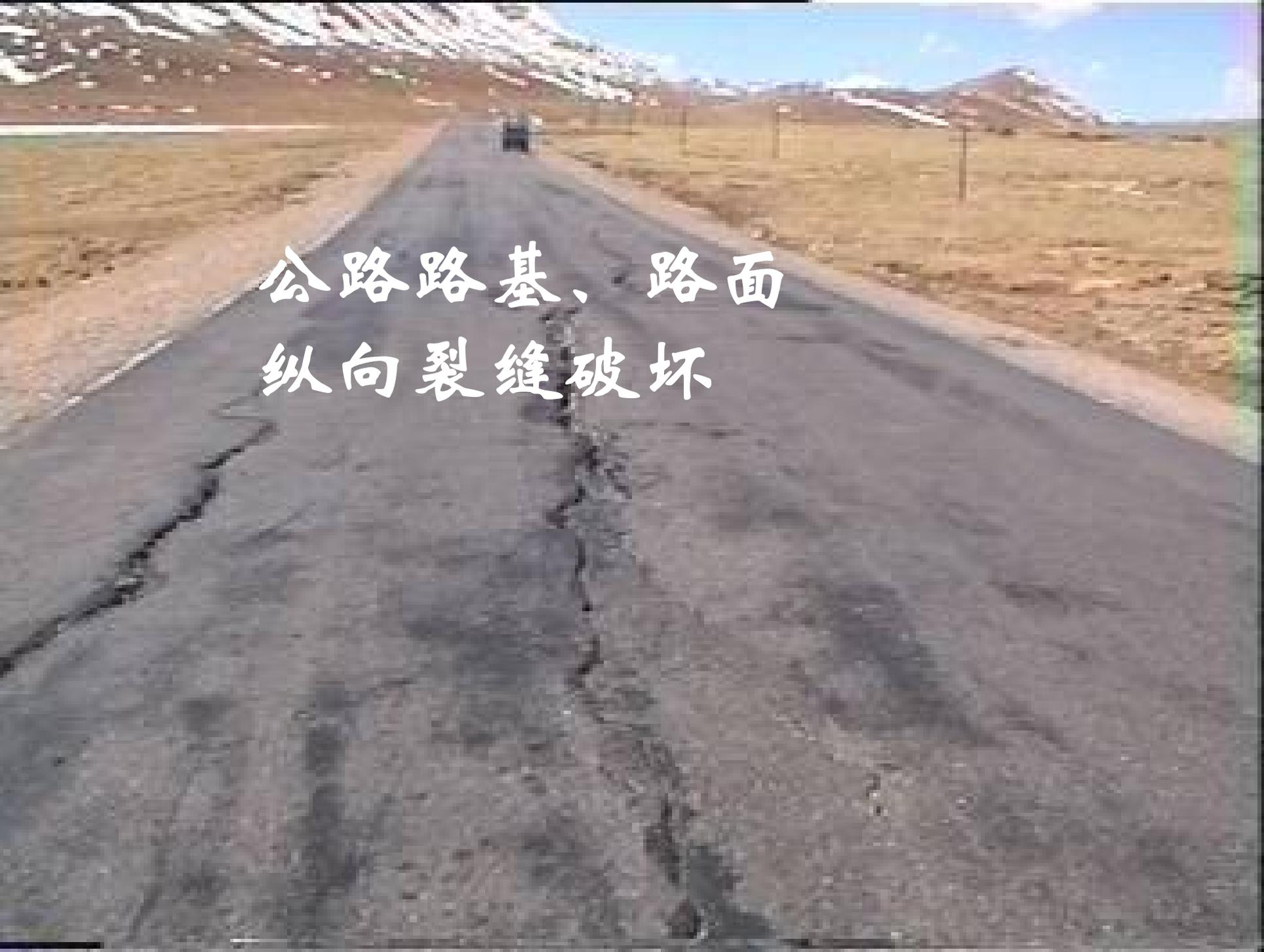
A photograph showing a road with significant longitudinal cracking in the pavement. The road is dark asphalt and runs through a dry, hilly landscape with sparse vegetation. The sky is blue with some clouds. The text is overlaid in the center of the image.
