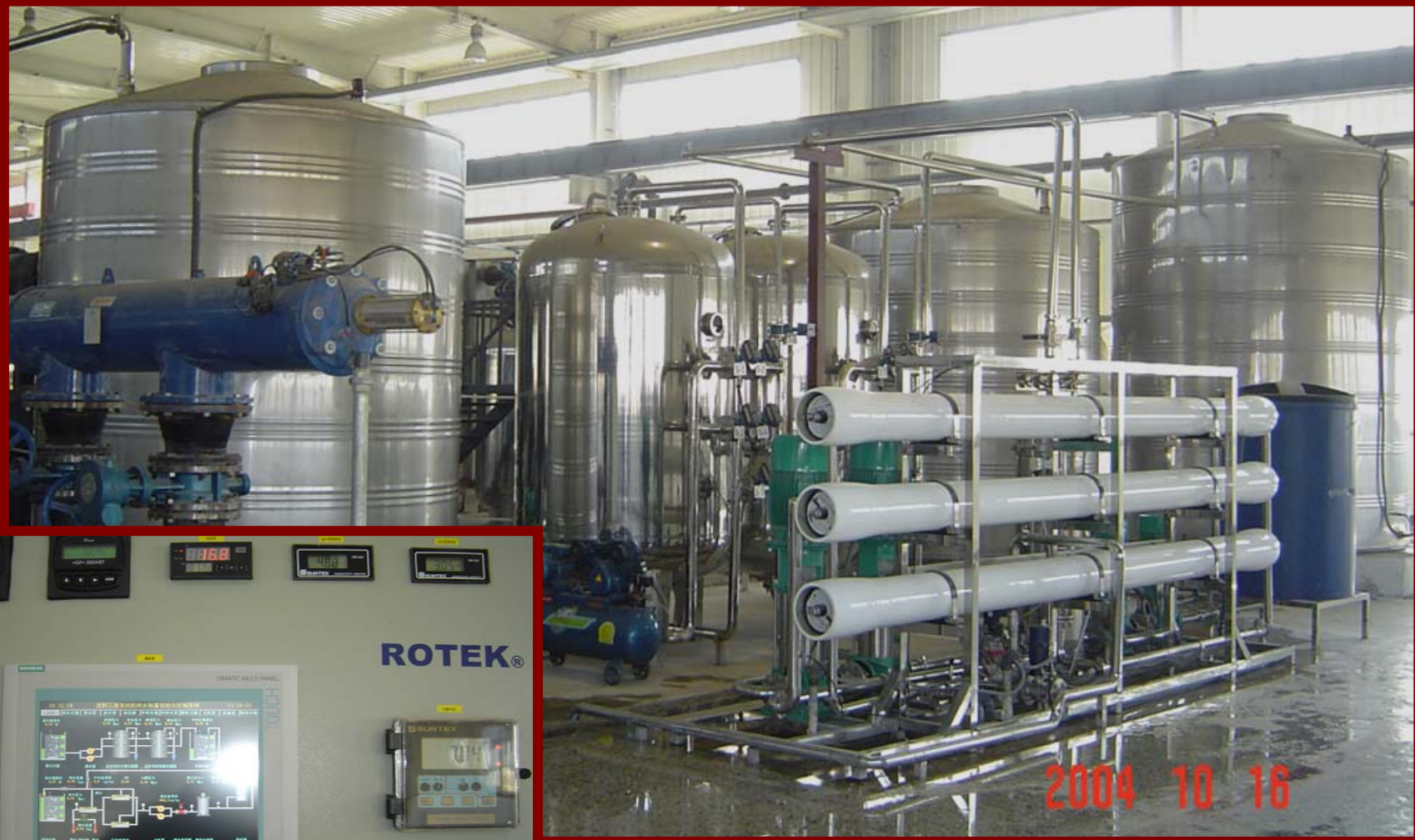
20 T/hr RO, Double Phase + Auto Mixing Beds with Multi-control Panel
