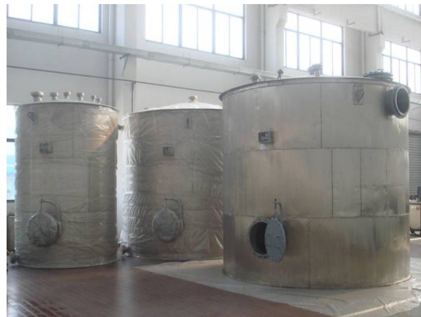
碱液循环槽 Anode Solution Tank
