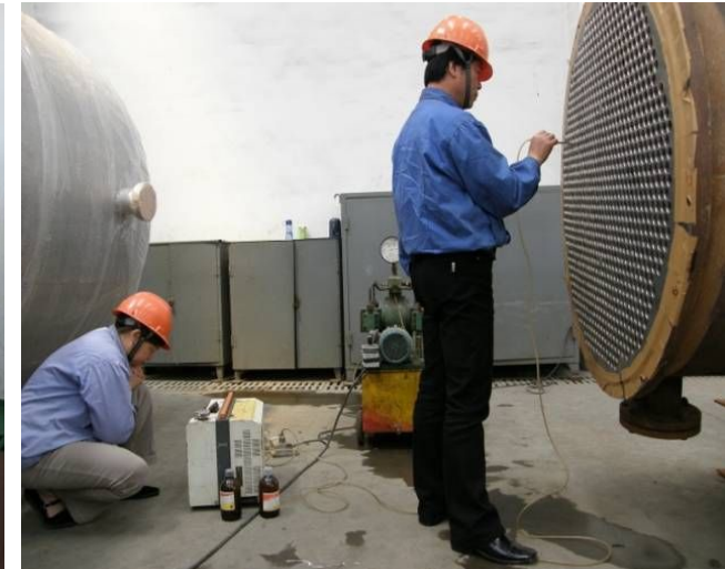
➤ 氦渗漏检测 Helium Leakage Test
