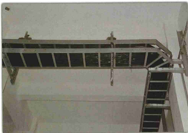
▲ Cable tray laying
