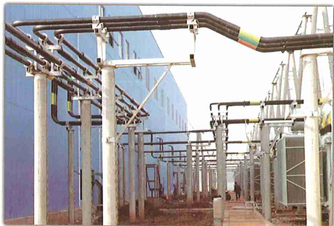
▲ Cable tube laying
