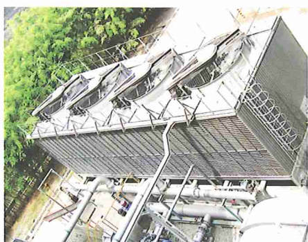
Cooling Tower for Condensate water
