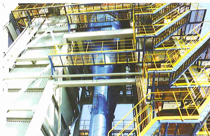
Hot Cyclone System of CFB Boiler 75ton 100bar 540°C
