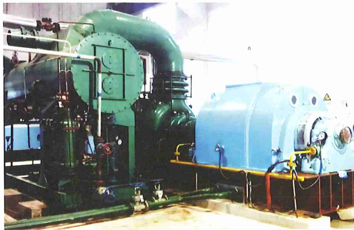
4500KW Extraction Condensing Turbine/Generator Boiler: 35ton 25bar 400°C Extraction for Process 15ton at 6 - 8bar
