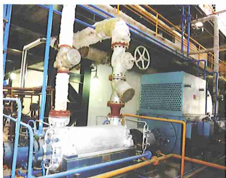
High Pressure Feed Water Pump
