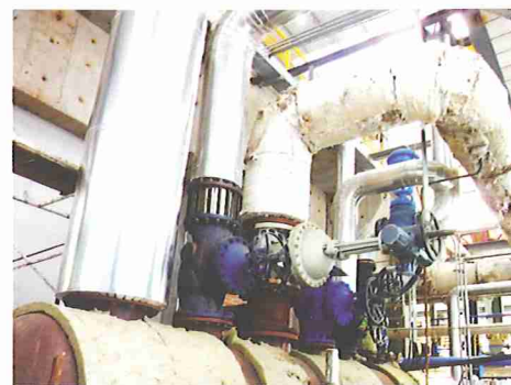
High Pressure Steam Header
