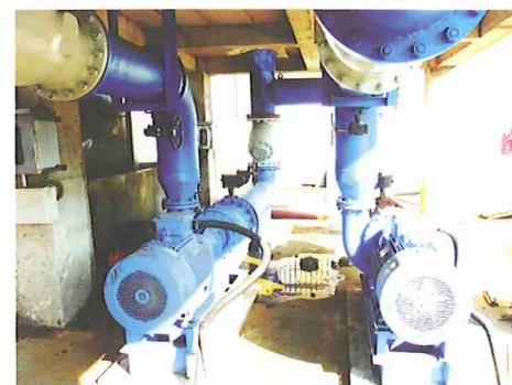
Cooling Tower Circulating Pump
